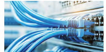
Altair Grid Engine significantly reduces overhead
