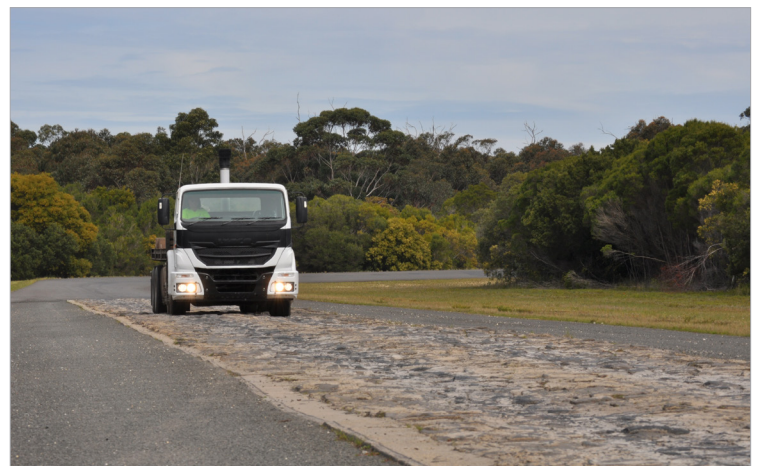
Belgian block paver test track
