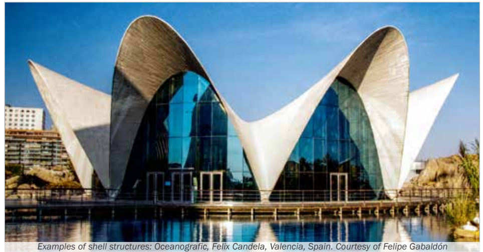
Examples of shell structures: Oceanographic, Felix Candela, Valencia, Spain. Courtesy of Felipe Gabaldón
