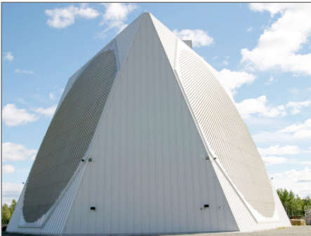
Fig. 01: Matrix of phased array antennas (AN/FPS-115 radar)
